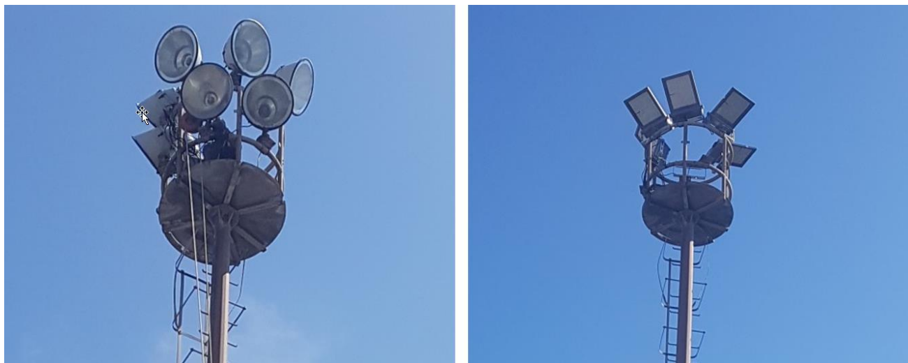
Figure 9: Old and new luminaires in the Port of Bar
