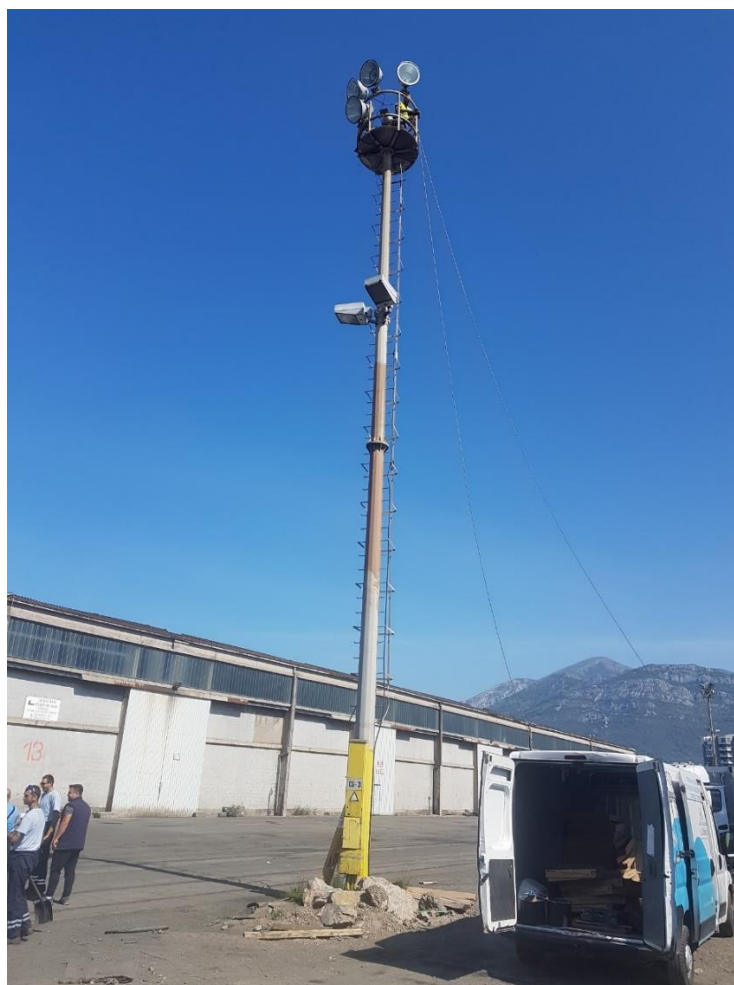
Figure 4: Old high-pressure sodium lamps prior the SMARTPORT pilot implementation
